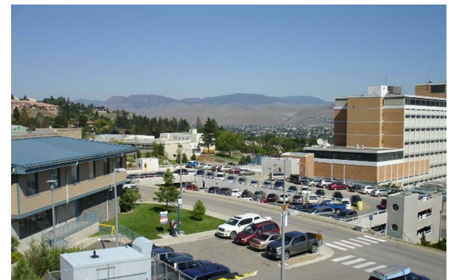
Existing Parking Deck Rear
