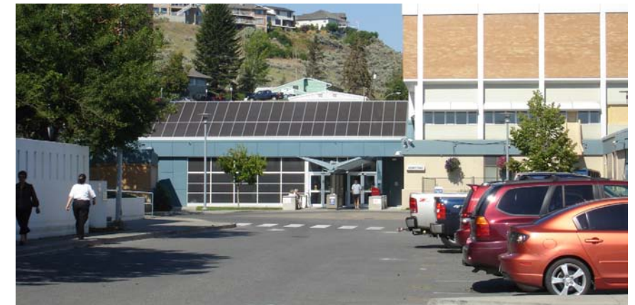
Existing Parking Main Entry
