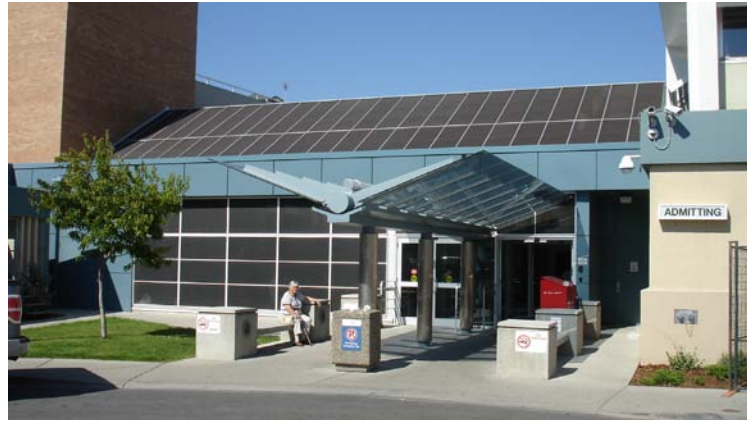
Main Entry and Drop-off
