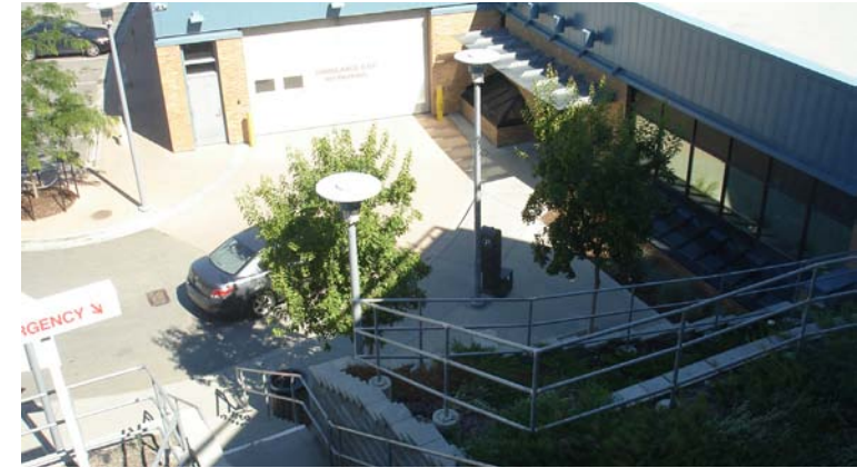
Ambulance Bay and Emergency Entrance
