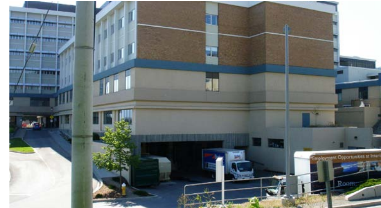
Main Building West Side Loading Area
